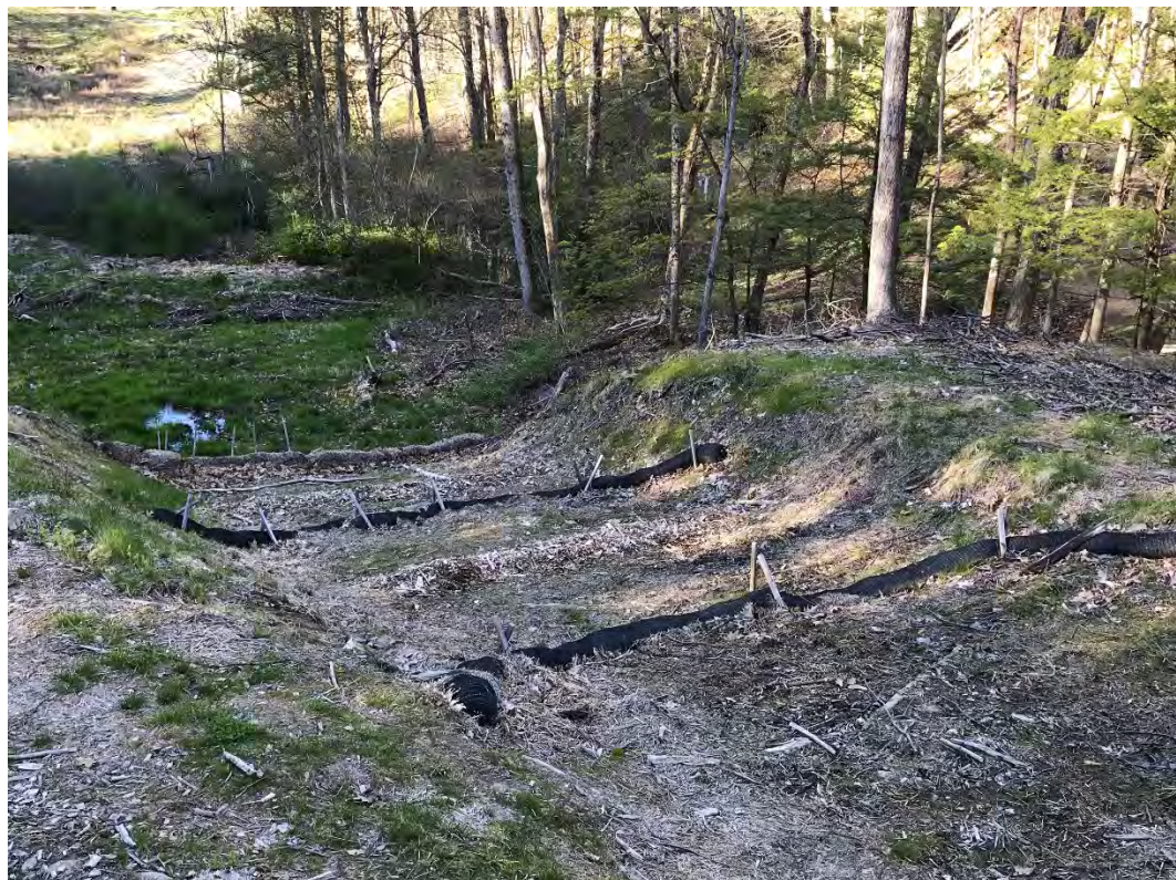
Fig 8: Lower portion of slope between Strs. 28 and 29. Viewing northeast. (05-06-21)
