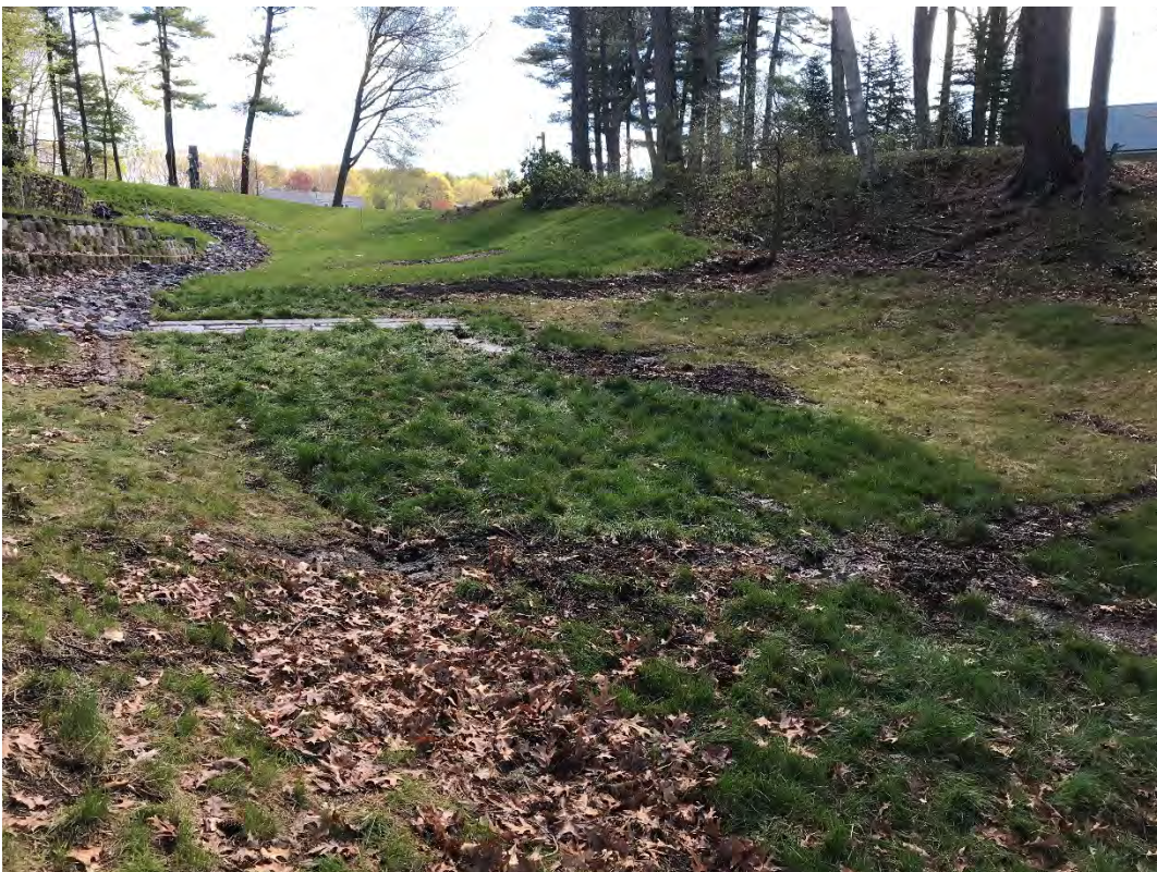
Fig 10: Slope below the manhole at Gundalow Landing/east side of the bay. Viewing east. (05-06-21)
