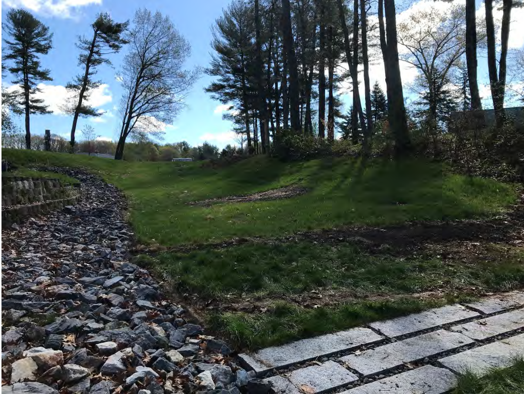
Fig 9: Slope above the manhole at Gundalow Landing/east side of the bay. Viewing east. (05-06-21)
