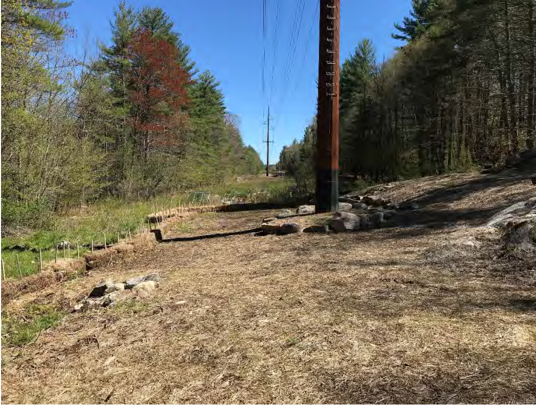
Fig 5: Str. 89 work area. Viewing southeast. (05-06-21)
