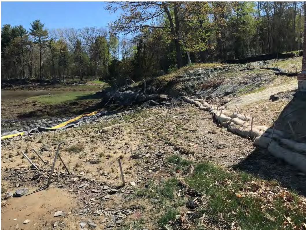
Fig 4: Toe of the slope and salt marsh restoration at the west side of the bay. Viewing south. (05-06-21)
